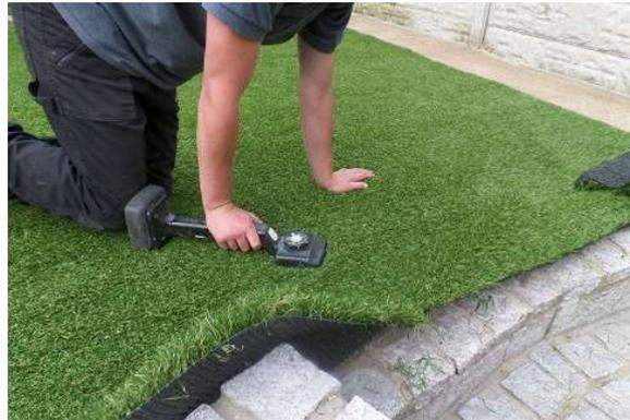
2.2 If the area that you are covering is wider or longer than the roll size (2m or 4m x 25m) you must take care to ensure that the pile of the adjoining piece runs in the same way as the first part. **This is very important.**
